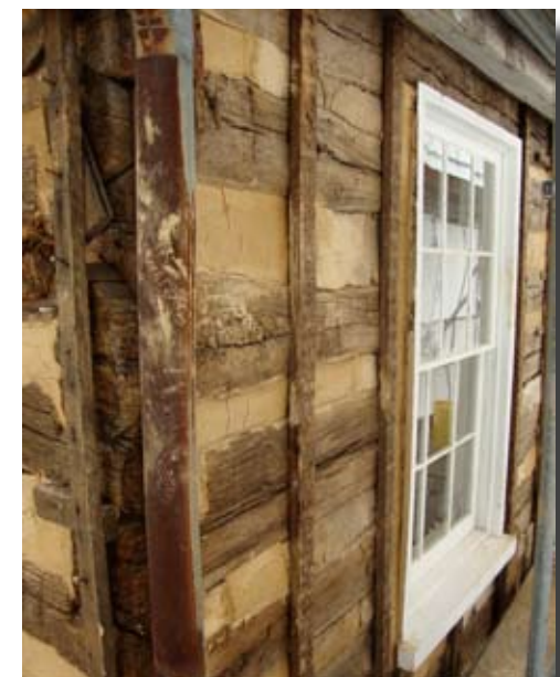
After the logs are repaired they are re-chinked.
